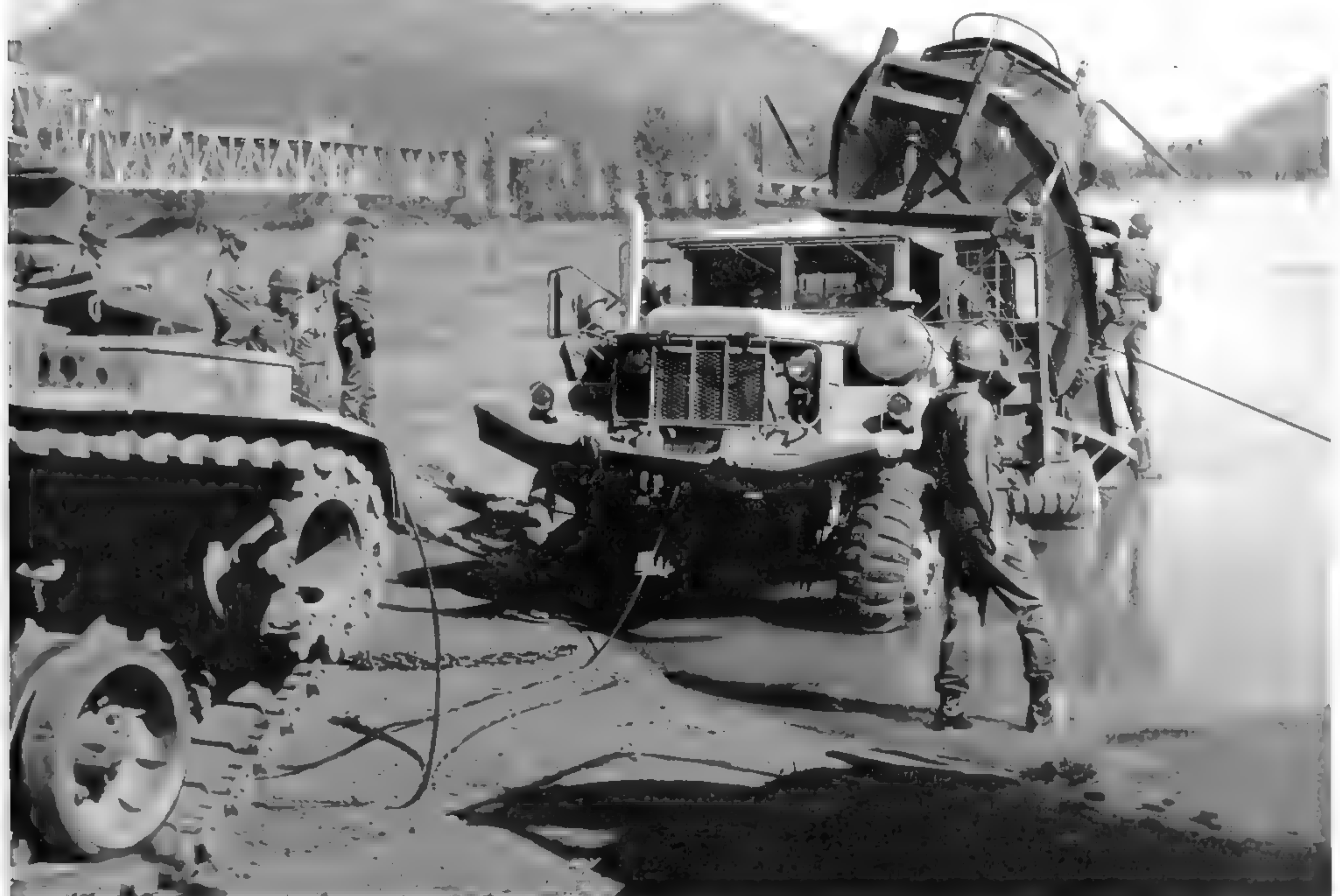
During bridge launch operations, the transporters were backed into the water, and the bridge sections expanded and launched, as seen here. (Photo courtesy of the Patton Museum)
